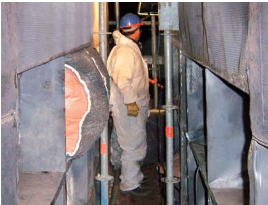
Exhaust splitter refurbishment.
