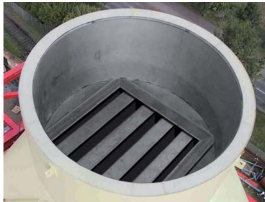
Exhaust stack with silencers.
