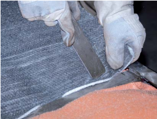
isoTECH® Compound installation.
