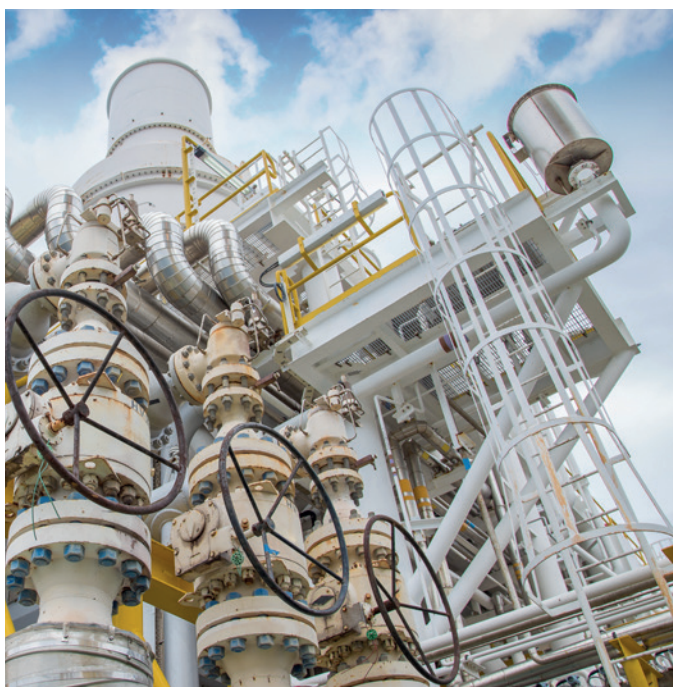
Plant turnaround: Every flange gasket needs to be replaced
