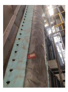
Challenging installation situation: The fabric expansion joint must be installed in a vertical duct. *Image:* © *Frenzelit GmbH*
