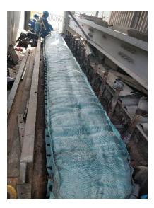
Precision-fit insulating packings are absolutely essential for the expansion joint at high temperatures because they lower the application temperature. *Image:* © *Frenzelit GmbH*
