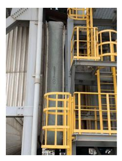
Ready for high temperatures, movements and expansion: The replaced fabric expansion joint with insulating layers made from high-temperature fibers by Frenzelit. Image: © *Frenzelit GmbH*
