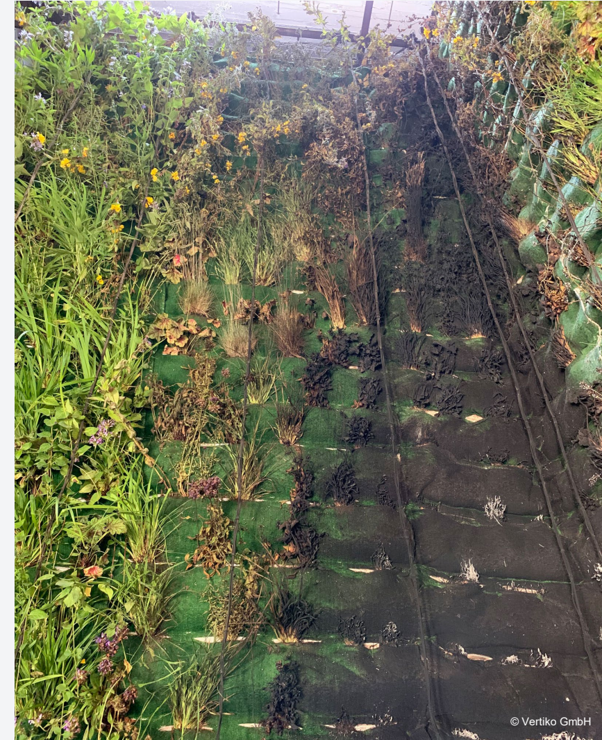
The image shows the result after a fire test.
